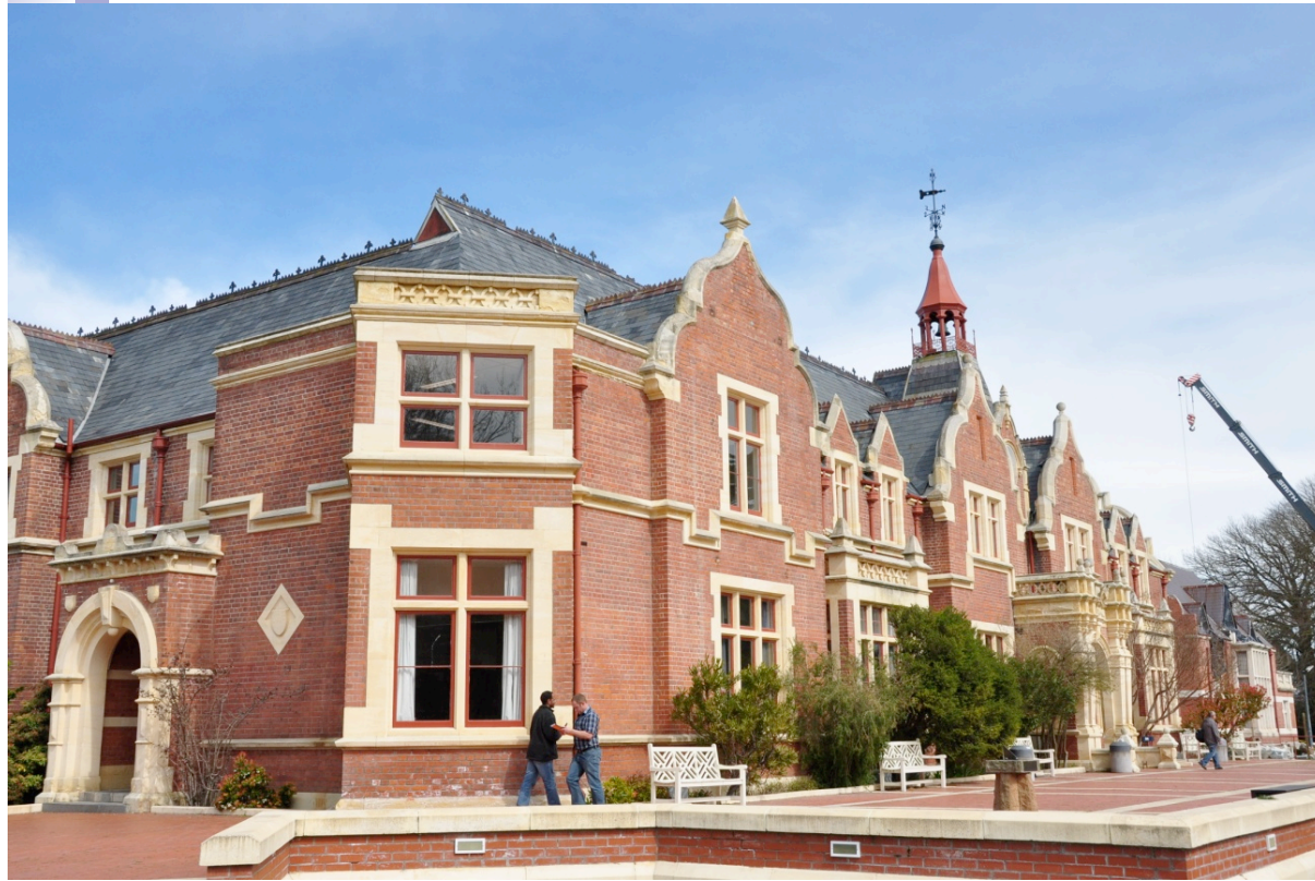
Ivey Hall Retrofitted
